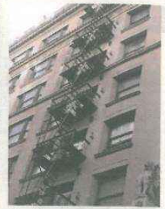
6 a fire escape
