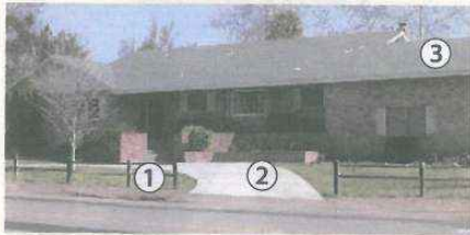
1 a fence 2 a driveway 3 a roof
